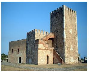
battery still face the river approaches. The central tower of the building is almost 60ft high, with walls over 6ft thick. The fortified walls around the building are almost 10ft thick, except on the river-side where the walls are 3 feet thick.<sup>[16]</sup> The cement holding the stoned walls together is a mixture of gypsum, clay, lime and the blood of animals. Spanish colonizers used enslaved Africans and indigenous people to build the fortress out of local coral stone.
